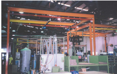
▲ Mobile Gantry Crane
