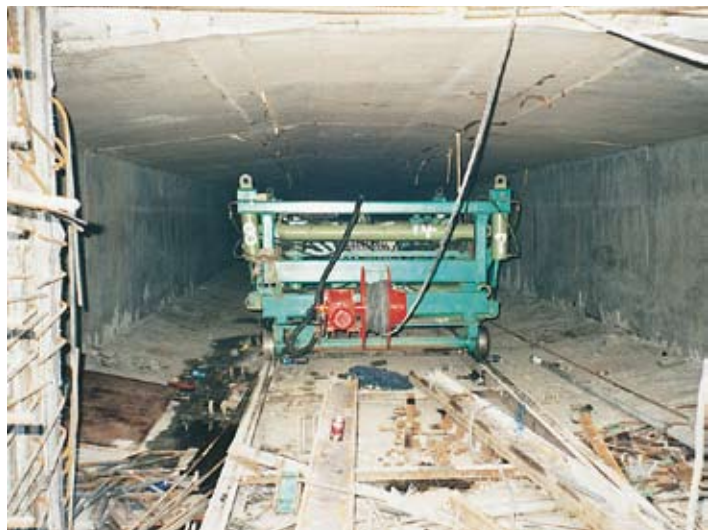
Civil Engineering: Cable In The Reinforced Concrete Box
