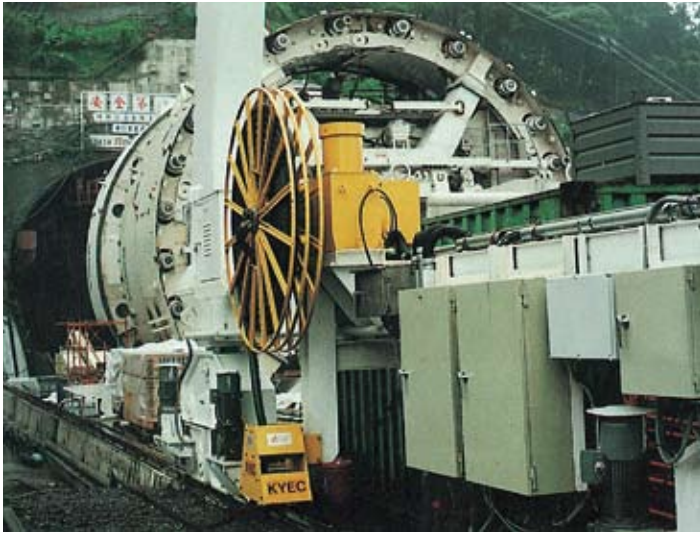
Tunnel Access 200 Ton Gantry Crane
